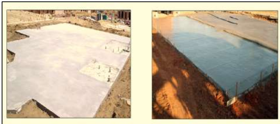
Figure 18: Raft or floating foundations which is convenient in construction site #1
